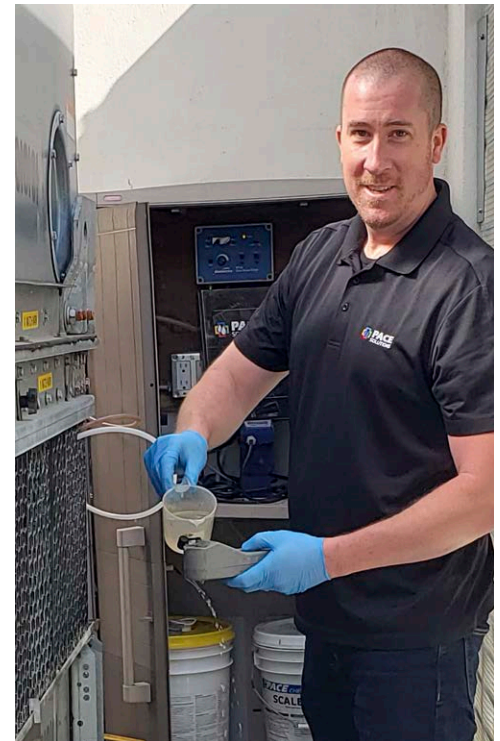
Mark Reid testing a fluid cooler in Vancouver.
